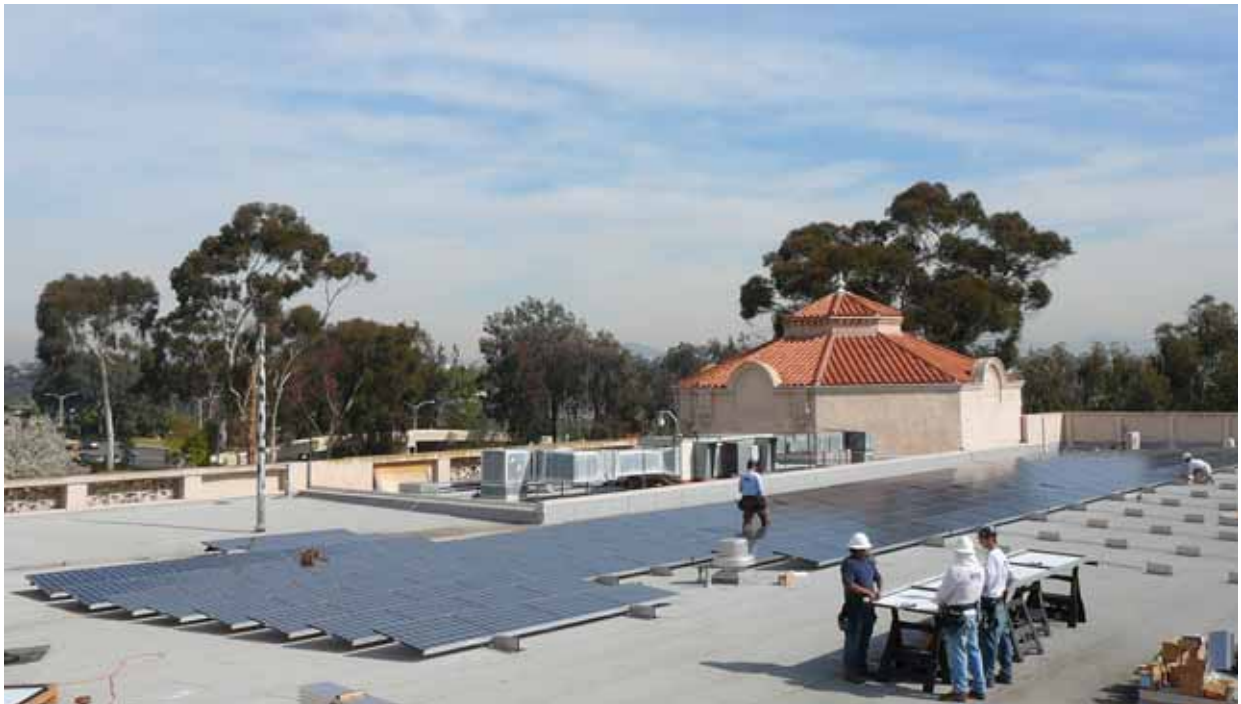
100kWac Commercial Install In Progress, Reuben H. Fleet, San Diego, CA
