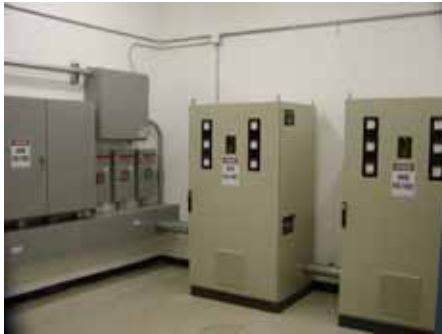
240 kWac PV/Diesel Hybrid – US Navy Site Santa Cruz Island
