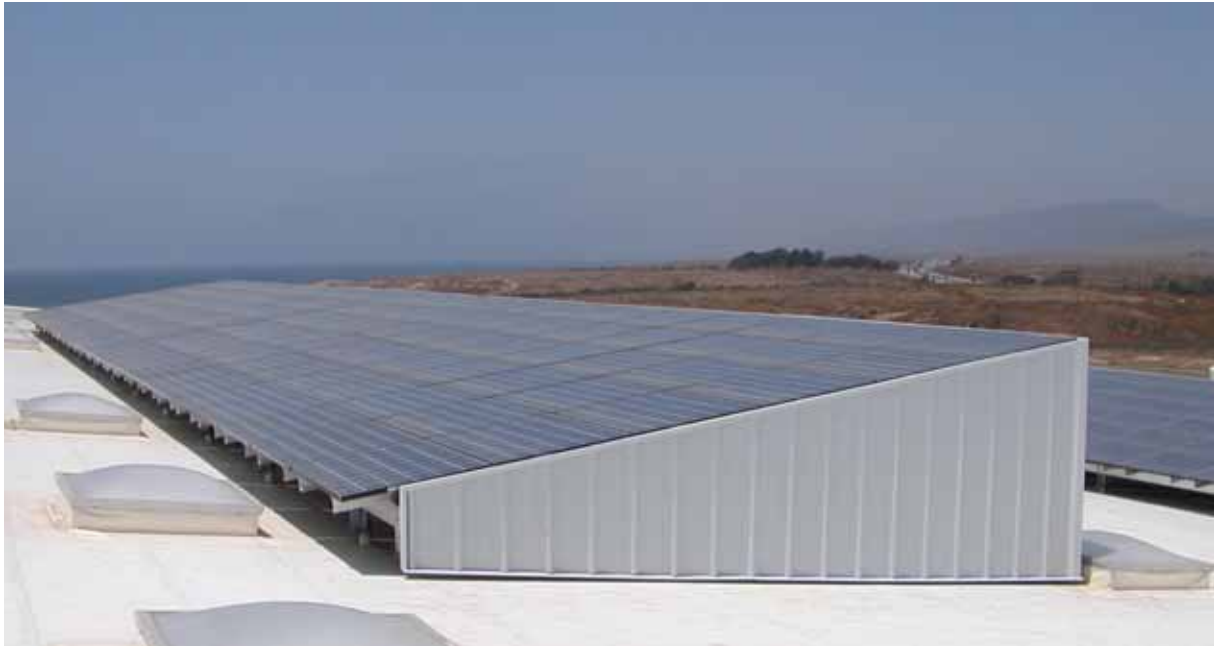
46 kWac Roof Mount – Camp Pendleton
